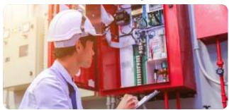
The Fire detection & Alarm Systems are conventional and addressable system. The detection fire fighting systems are divided into zones depending upon the nature of fire or hazard area. The detection fire fighting systems also contain manual push buttons sounders and flashers that activated a few second before the system to alert the occupants from fire.
