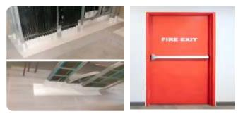
A passive protection system is a type of safety mechanism or feature designed to provide protection without requiring any active intervention or control. It typically operates automatically or passively in response to specific conditions or events, providing a level of protection without relying on human input or power sources.
