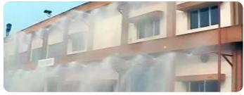
A drencher system can be installed in a podium, which is a structure that serves as a base for a building or a section of a building. In fact, a drencher system is often installed in the podium of high-rise buildings to provide fire protection to the lower floors of the building.
