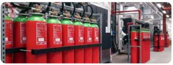
The Co2, Argon, HFCs, FM200 & high pressure water mist are used in these kind of fire fighting systems. The extinguishing agent is kept in cylinders at high pressure. The fire extinguishing fire fighting system is controlled by pilot cylinder or control valve by fire control panel via heat detectors or smoke detector or multisensory detector depending upon the nature of hazard area.
