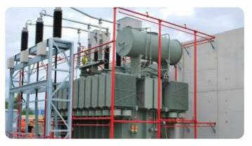
HVWS stands for High Velocity Water Spray System. It is a type of fire suppression system commonly used in industrial settings, such as power plants, chemical plants, and storage facilities. HVWS systems are designed to quickly extinguish fires that involve flammable liquids or gases.
