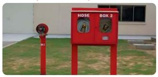
Water Hydrant Fire Fighting System consist of hydrants attached to same pipeline, the other end of the pipeline is attached to the pumps and water supply tank. The fire fighting hydrant line is close loop pipe system to maintain the pressure in the water hydrant fire fighting system. In Water Hydrant Fire Fighting System hydraulic calculations are done according to NFPA standards.
