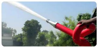
Water / Foam Monitor Fire Fighting System works same as Water Hydrant Fire Fighting System instead of hydrants fire monitors are installed on the fire fighting pipeline. Fire monitor fire fighting systems are installed on open type hazards. Fire monitors has high velocity nozzles attach to the end of the pipe which laminate the water steam and project it at a long distance more than 100 feet.
