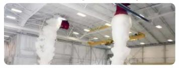
A water foam sprinkler system is a type of fire suppression system that uses water and foam to extinguish fires. The system is composed of a network of pipes, sprinkler heads, and a foam concentrate storage tank.
