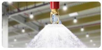
Water / Foam Sprinkler Fire Fighting System consists of fire sprinklers attached to the fire fighting pipeline and are installed at the top on ceiling or on the wall. The water sprinkler fire fighting system may be wet type of dry type depending upon the temperature and distance of fire fighting water source from the hazard and nature of fire hazard.
